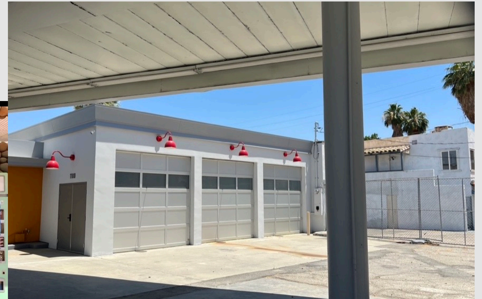
Potential location near downtown Palm Springs, former service station on Palm Canyon Drive.
